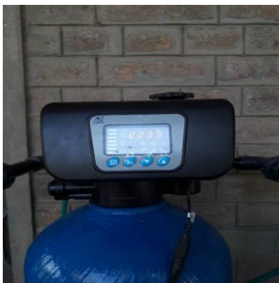
Figure 7: Multi-Functional Flow Control Valve for Water Treatment
