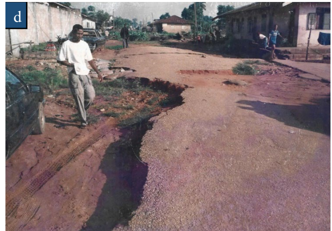
Figure 2: Pictures of environmental degradation by gully erosion in Benin City. (a) Destruction of houses and groundwater pollution from leachate from refuse at Constain road, New Benin, (b) Loss of soil behind Uniben, Ugbowo, (c) and (d) Loss of soil and truncation of roads behind Queen Ede School, Ikpoba Hill.
